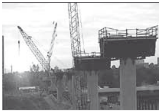
DC Metro construction
