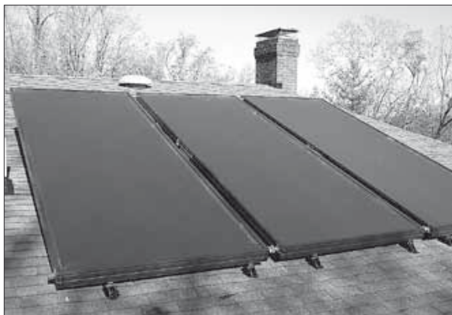
Solar panels on roof of Jablonski home heat the household water most of the year.
