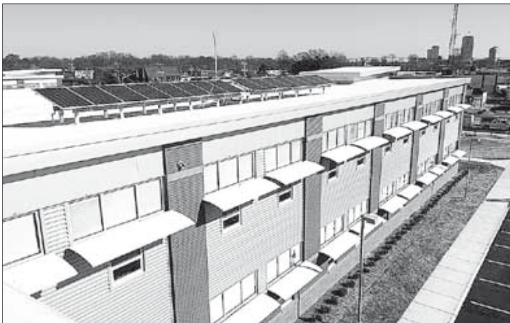
Metal shelves on brackets below the windows reflect light into the classrooms. Solar panels on the roof heat water for the school's kitchen.
