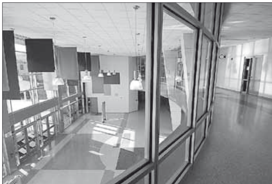
Daylight coming into the two-story windows in the front hallway provides light back into the building on two floors.
